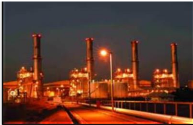
Sta Rita Natural Gas-fired Plant
