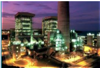
1294 MW Sual Coal-fired Power Plant
