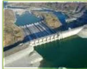
360 MW Magat Hydroelectric Power Plant
