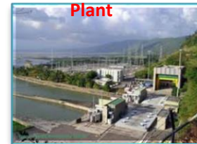
755MW CBK Hydroelectric Power Plant
