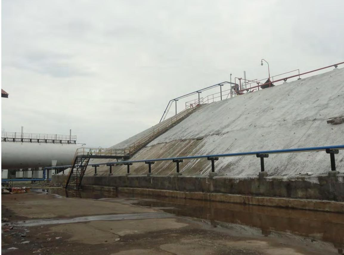
**ABOVE GROUND TANKS and MOUNDED TANK in one LOCATION**
