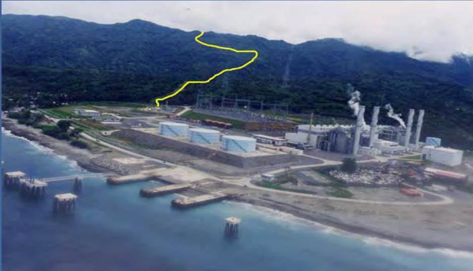
From the 1200 mw Ilijan Combined Cycle Power Plant
