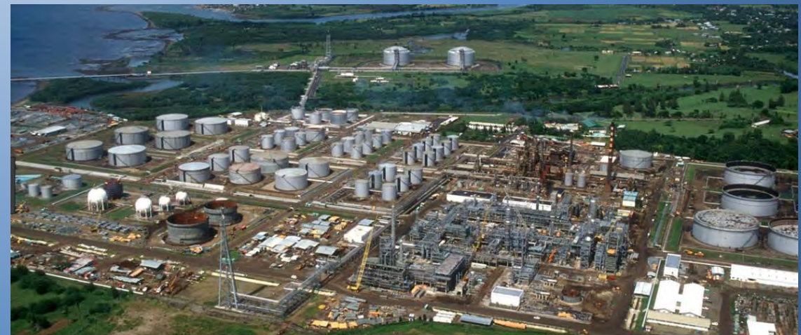
Malampaya Onshore Gas Plant, Tabangao, Batangas City
