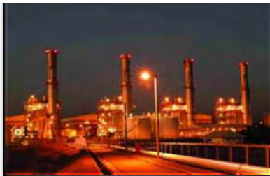
Sta Rita Natural Gas-fired Plant
