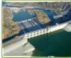
360 MW Magat Hydroelectric Power Plant
