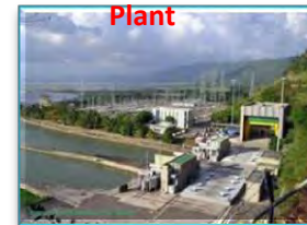
755MW CBK Hydroelectric Power Plant
