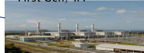
1,000 MW Sta. Rita First Gen/ IPP
