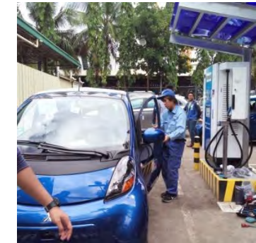
Use of FAST Electric Vehicle Charger will encourage use of EV for cleaner alternative
