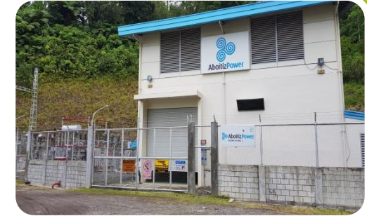
6.6MW Tudaya 1 Hydroelectric Power Plant in Sta. Cruz, Davao del Sur
