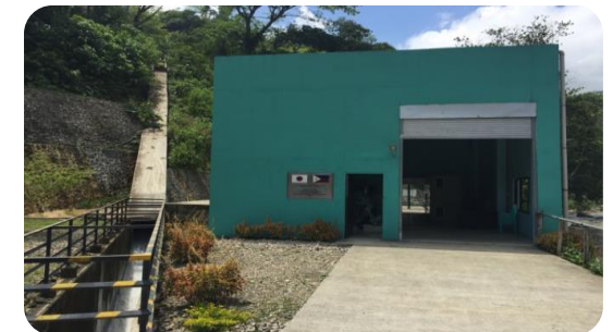
0.82MW Likud Hydroelectric Power Plant in Asipulo & Kiangan, Ifugao
