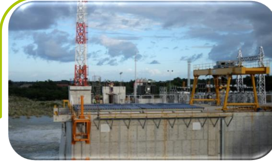
8.50MW Maris Main Canal 1 Hydroelectric Power Plant in Ramon, Isabela
