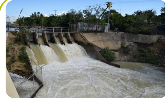
1.0MW Prismc Hydroelectric Power Plant in Rizal, Nueva Ecija
