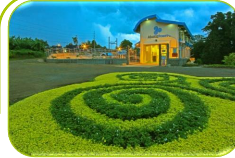
7.0MW Tudaya 2 Hydroelectric Power Plant in Sta. Cruz, Davao del Sur
