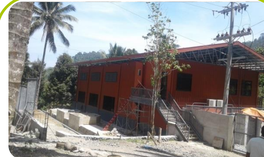
3.0MW New Bataan Hydroelectric Power Plant in New Bataan, Compostela Valley
