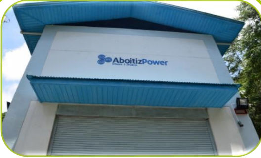
3.80MW Irisan 1 Hydroelectric Power Plant in Tuba, Benguet
