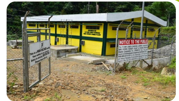
3.0MW Linao-Cawayan (Upper Cascade) Hydroelectric Power Plant in San Teodoro, Oriental Mindoro
