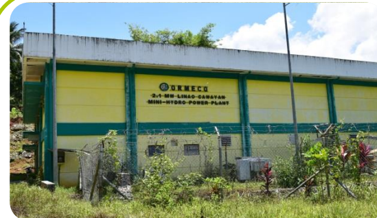
2.1MW Linao-Cawayan (Lower Cascade) Hydroelectric Power Plant in San Teodoro, Oriental Mindoro
