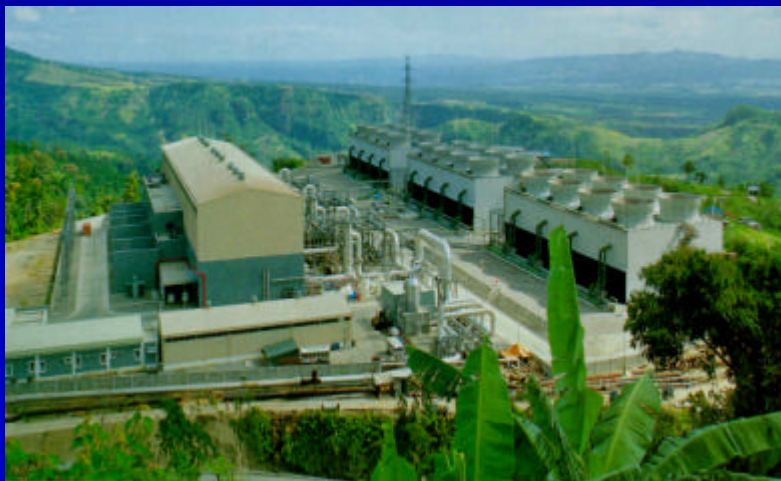
Malitbog Facility in Leyte: Largest Geothermal Power Plant in the World
