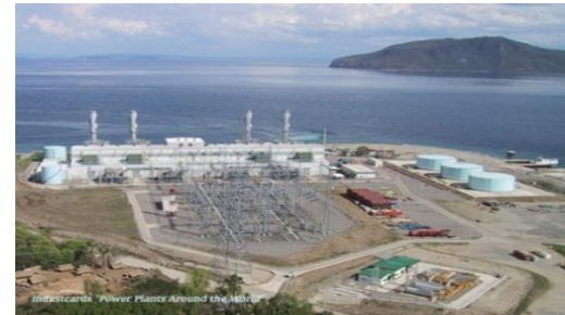
1,200 MW Ilijan Power Plant NPC IPP(KEPCO)
