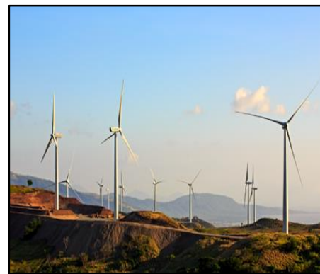
Pililla Wind Farm (Rizal)
