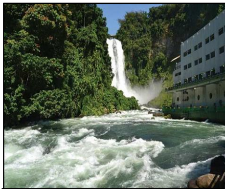
AGUS VI Hydroelectric Power Plant (Iligan)
