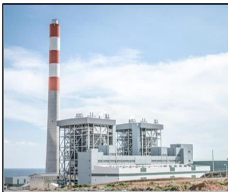
GNPower Mariveles Coal-Fired Power Plant (Bataan)
