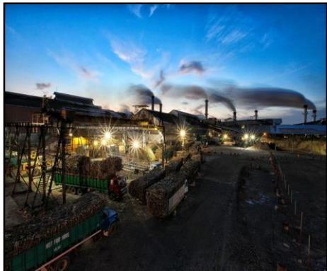
VMC Bagasse-fired Cogeneration Plant (Negros)
