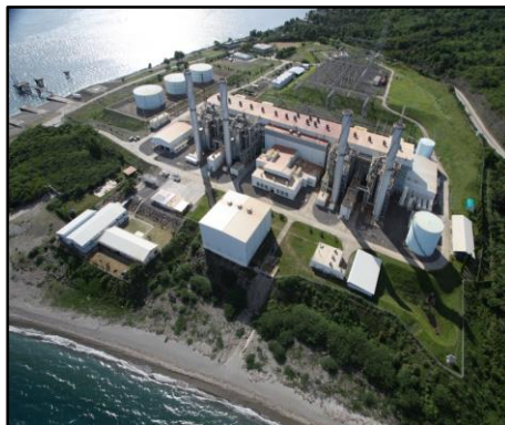
Ilijan Combined-Cycle Power Plant (Batangas)
