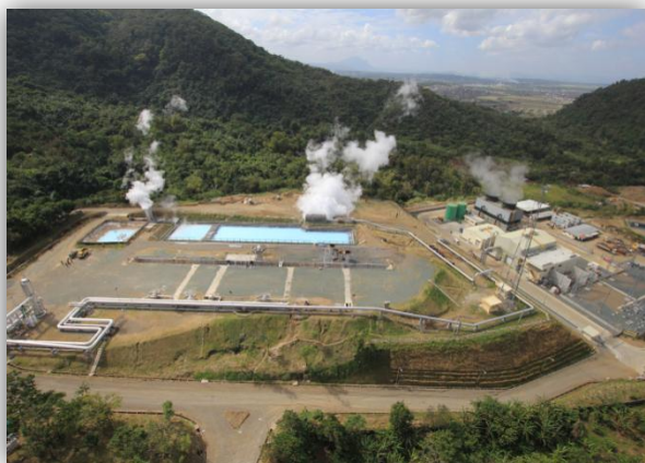
The 20-MW Maibarara Geothermal Power Project started commercial operations on 08 February 2014 (Photo courtesy of Maibarara Geothermal, Inc.)
